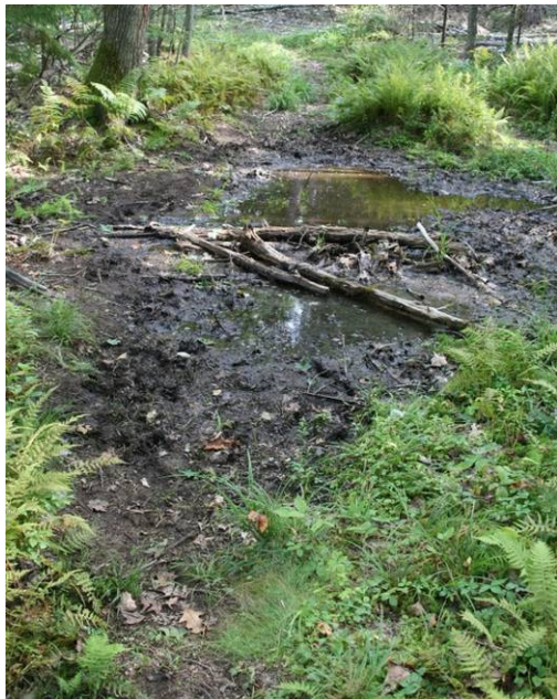
Figure 2 A wet and muddy section of trail. Note the wet and muddy area is wider than nearby trail segments, has bare soil, and embedded footprints.
